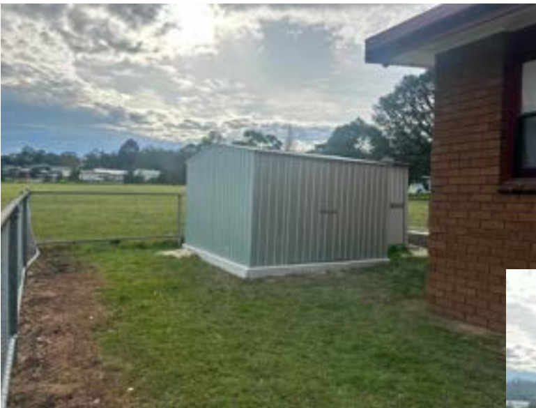
Brand new shed, ready for service!
